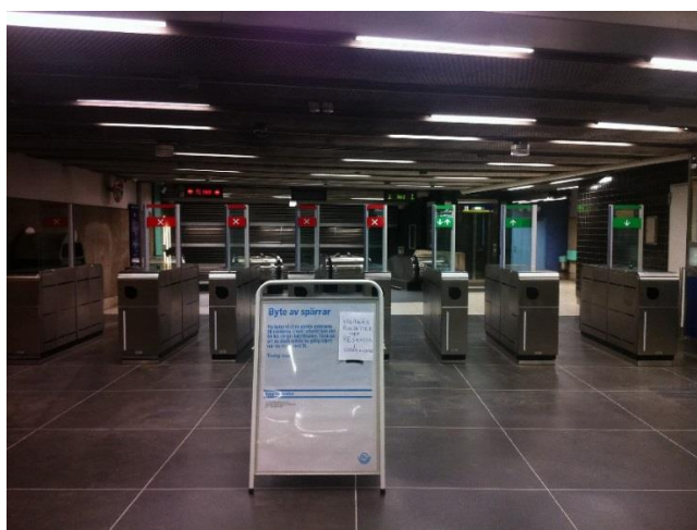
Figure 12. Replacement of barriers at the Stadion metro station. Photo: by the author.
